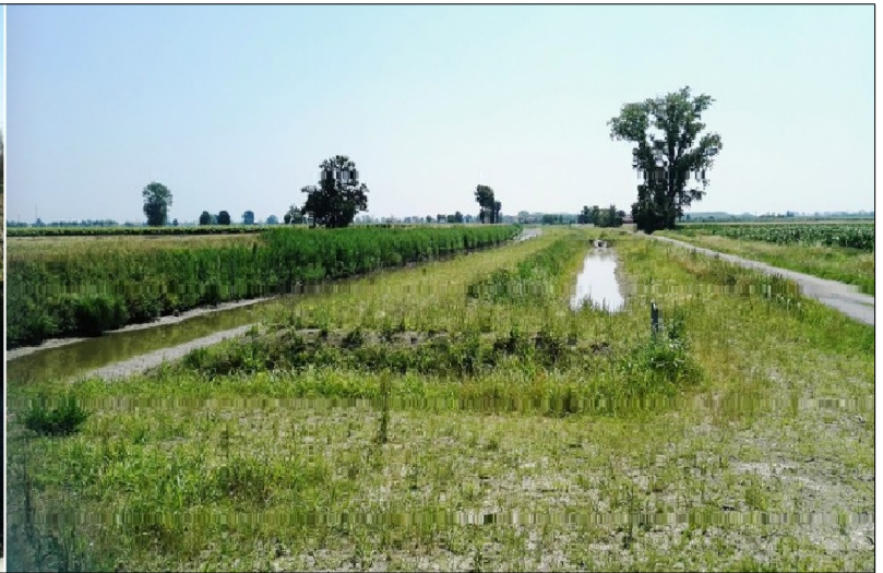
Collettore Alfieri canal after works (june, 2016)
